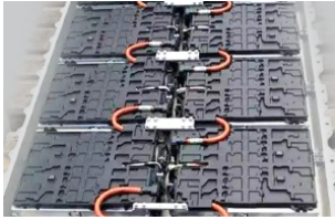
Battery charge/discharge test
